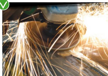
FLATTENING OF WELDING RIDGES
