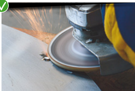
REMOVAL OF IMPERFECTIONS
